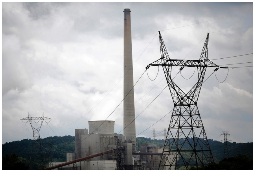
Appalachian Electric Power's coal-fired Big Sandy Power Plant, Cattlesburg, Ky
