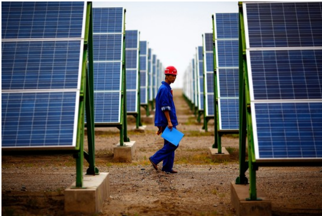
A worker inspects solar panels in Dunhuang, China. We have an estimated supply of one million years of tellurium, a rare element used in some panels.
