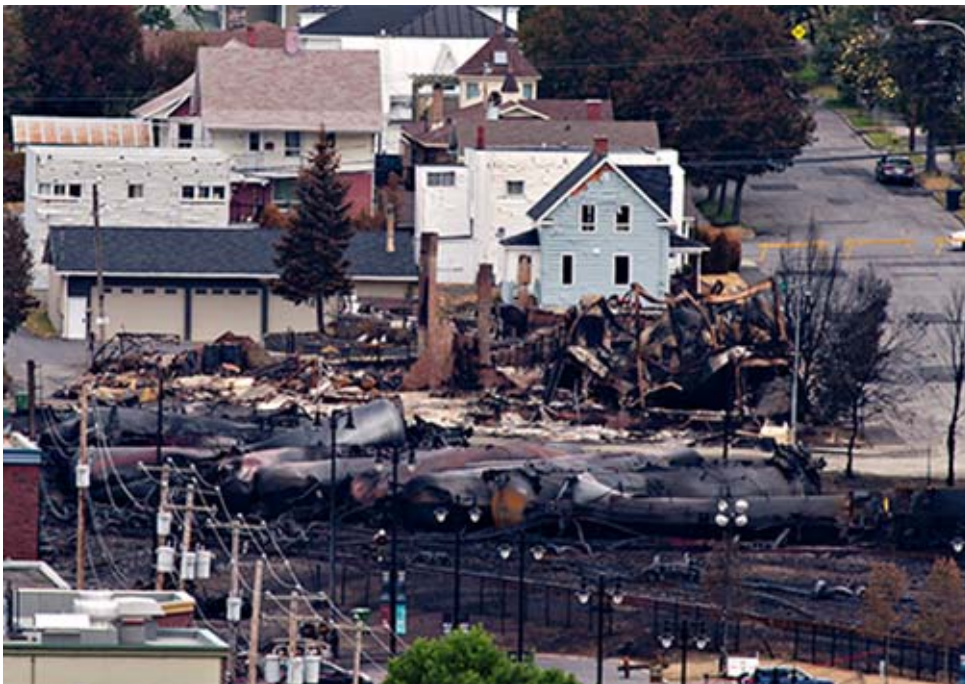
Charred tanker cars are piled up in Lac-Megantic, Quebec
