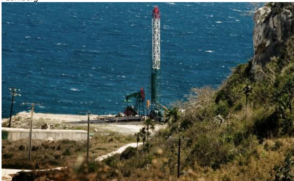
An oil and gas pumping station in Santa Cruz, east from Havana, Cuba.
